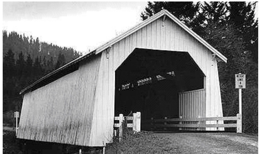
Hayden Bridge, Benton County
