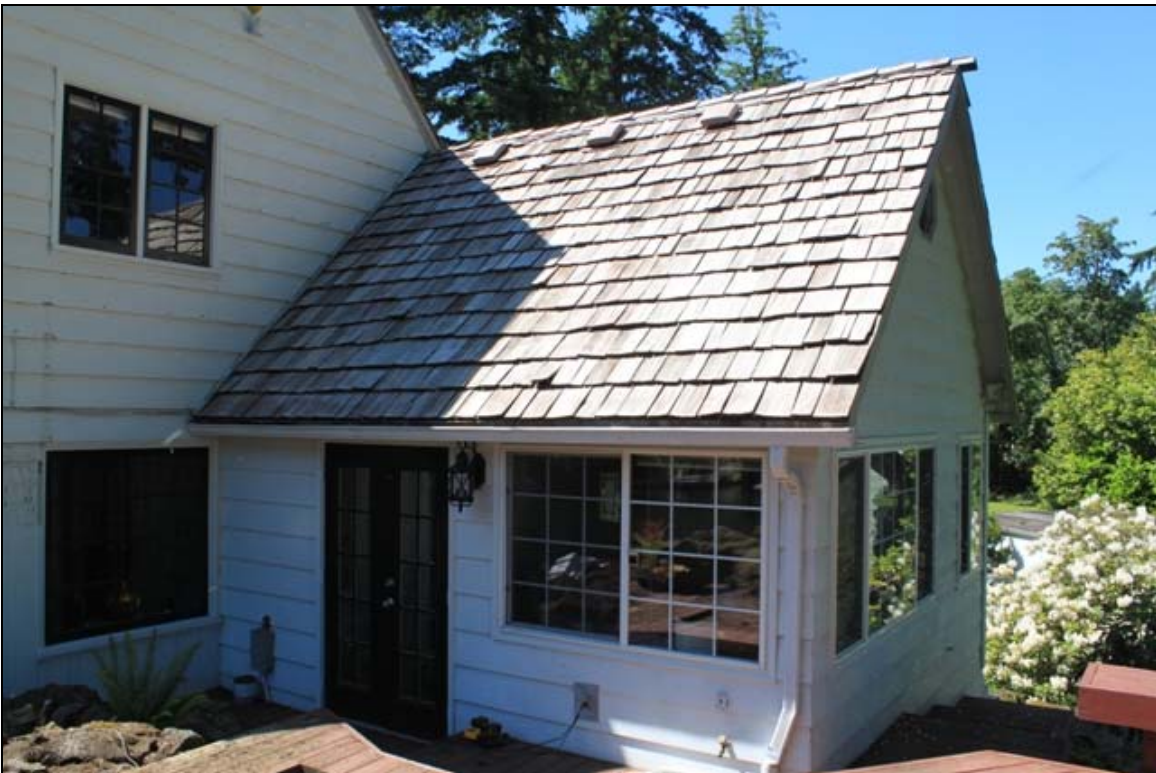
Photo 2 of 15: (OR_ClackamasCounty_OscoC.RoehrHouse_0002) East façade, camera facing northwest
