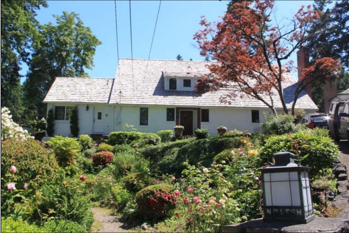
Photo 1 of 15: (OR_ClackamasCounty_OscoC.RoehrHouse_0001) North façade, camera facing south
