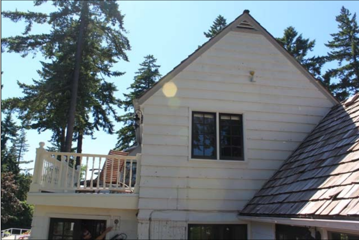
Photo 3 of 15: (OR_ClackamasCounty_OscoC.RoehrHouse_0003) East façade, camera facing west, second floor
