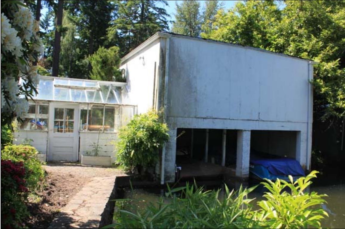
Photo 7 of 15: (OR_ClackamasCounty_OscoC.RoehrHouse_0007) Boathouse, camera facing north
