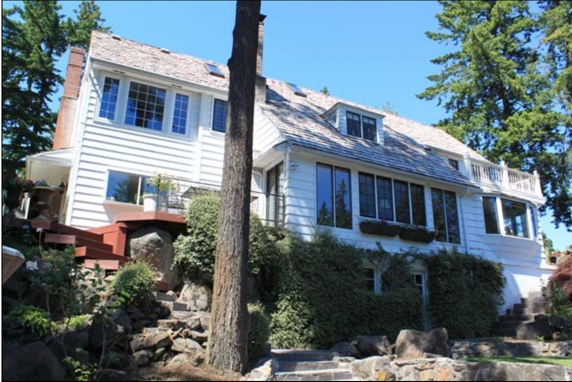
Photo 5 of 15: (OR_ClackamasCounty_OscoC.RoehrHouse_0005) South façade, camera facing northeast
