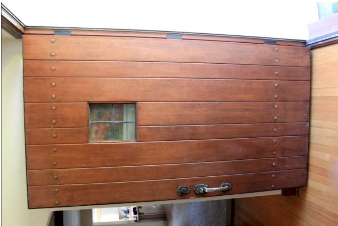
Photo 8 of 15: (OR_ClackamasCounty_OscoC.RoehrHouse_0008) Front door detail, camera facing west
