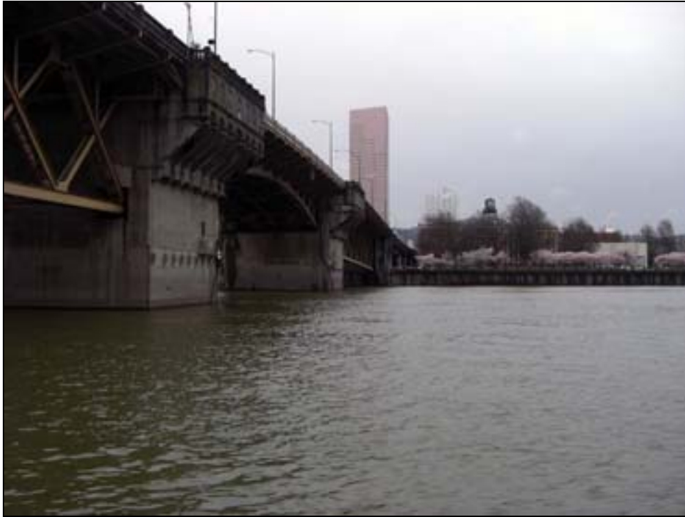
Photo 3 of 6: (OR_MultnomahCounty_WillametteHwyBridgesMPD_BurnsideBridge_0003) Downstream view, looking west, toward downtown Portland, from Vera Katz Esplanade
