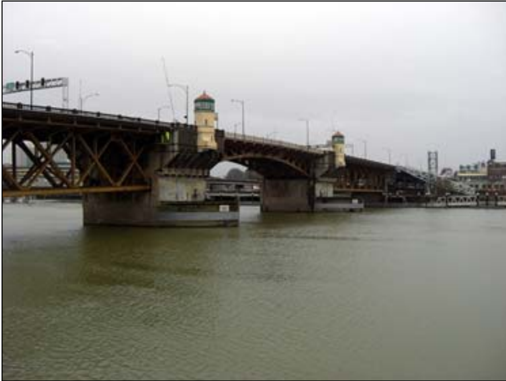
Photo 1 of 6: (OR_MultnomahCounty_WillametteHwyBridgesMPD_BurnsideBridge_0001) Upstream view, looking NE, from west side bike path
