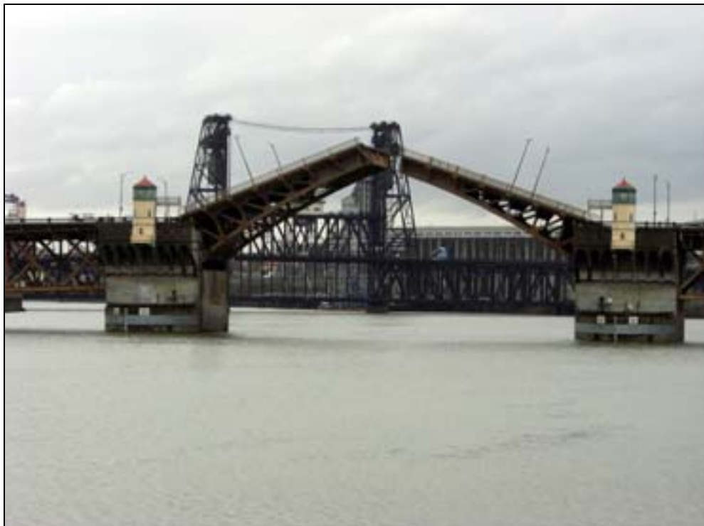
Photo 6 of 6: (OR_MultnomahCounty_WillametteHwyBridgesMPD_BurnsideBridge_0006) Downstream view, showing bascule in operation (Steel bridge in distance)
