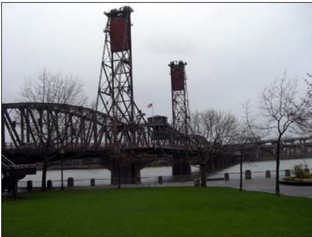
Photo 2 of 5: (OR_MultnomahCounty_WillametteHwyBridgesMPD_HawthorneBridge_0002) Upstream General View, Looking E, from McCall Park
