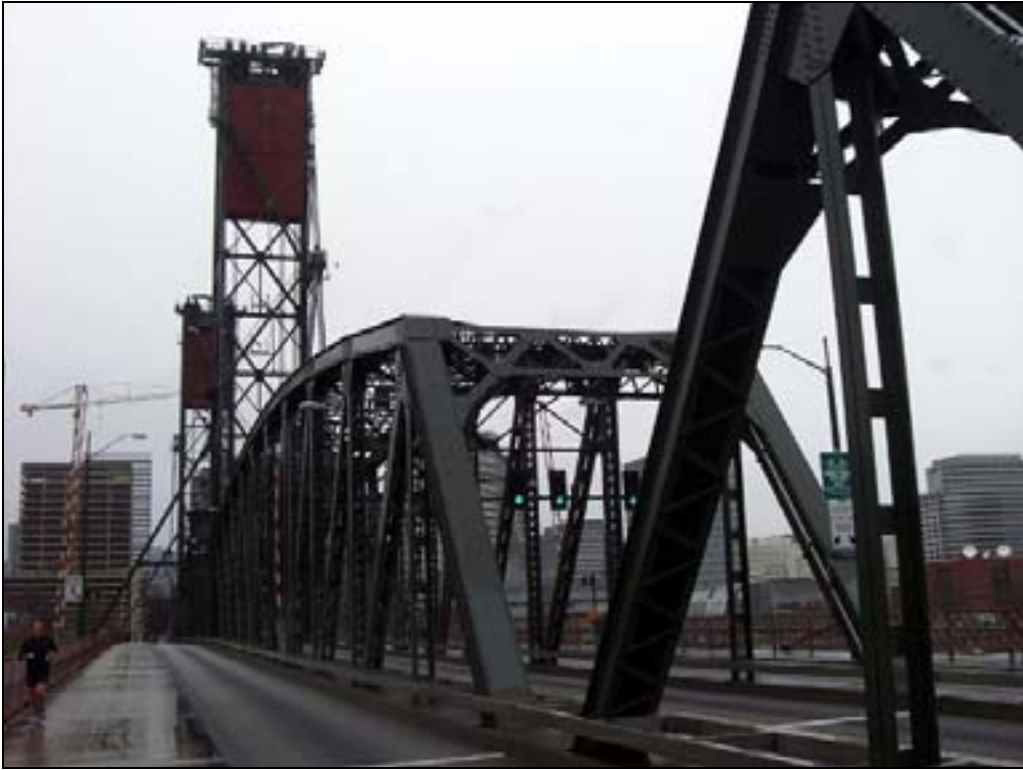
Photo 3 of 5: (OR_MultnomahCounty_WillametteHwyBridgesMPD_HawthorneBridge_0003) On bridge, looking west, toward downtown
