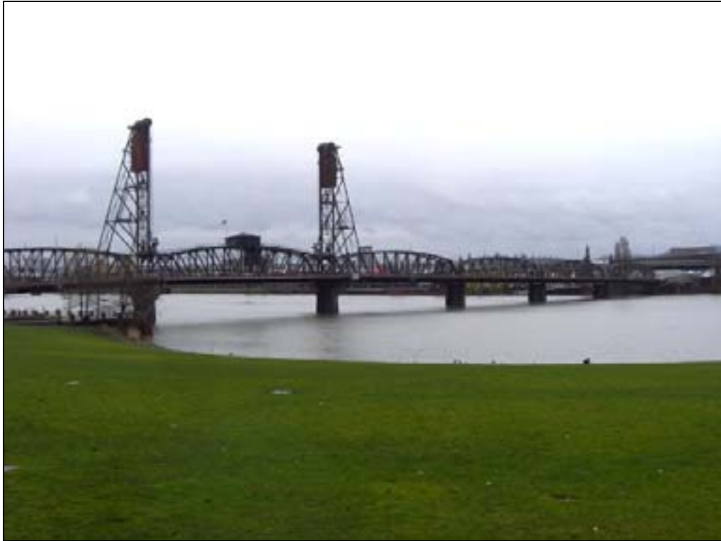
Photo 1 of 5: (OR_MultnomahCounty_WillametteHwyBridgesMPD_HawthorneBridge_0001) General View, Looking Upstream (NE) from McCall Park
