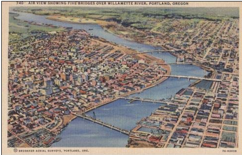
Figure 5: Five Bridges Over the Willamette River, looking north, c. 1927 author's collection, Hawthorne Bridge at bottom of image
