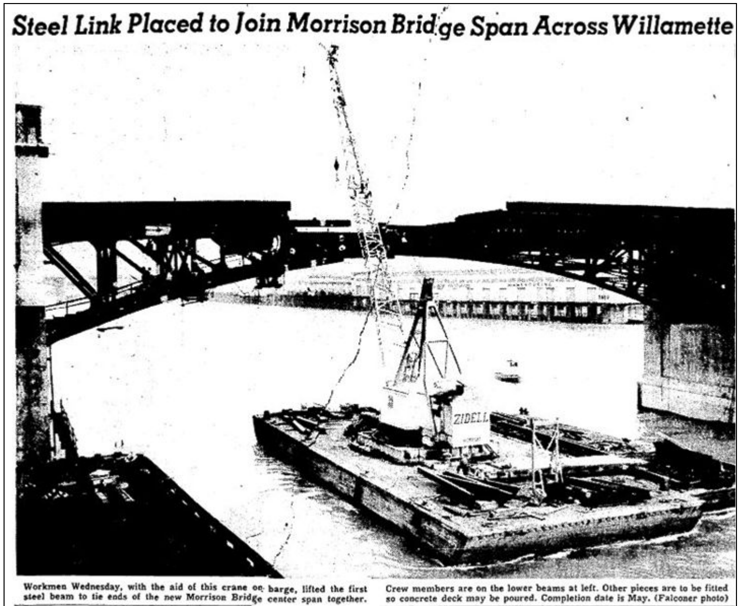
Figure 7: Newspaper Excerpt, Steel Link Placed to Join Morrison Bridge Span Across the Willamette Oregonian , 20-February-1958, 5:1-5
