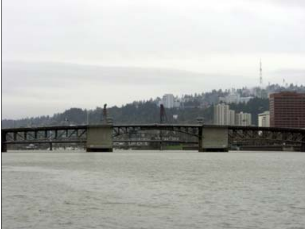
Photo 1 of 5: (OR_MultnomahCounty_WillametteHwyBridgesMPD_MorrisonBridge_0001) General View, Looking Downstream, from the Hawthorne Bridge
