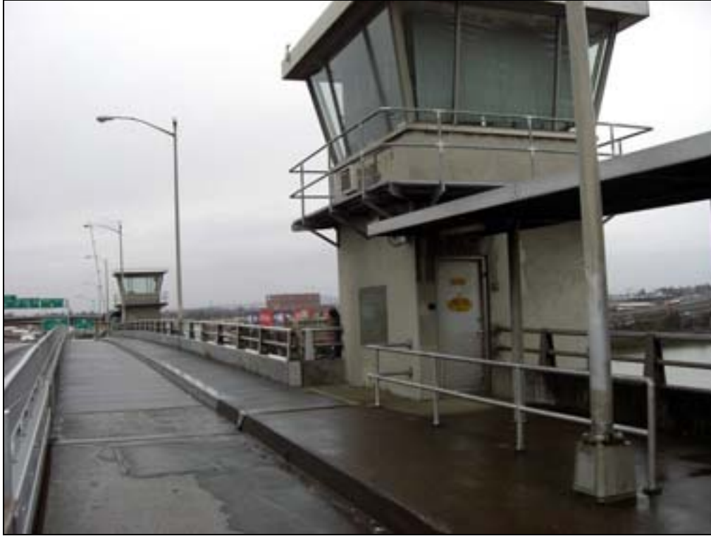
Photo 4 of 5: (OR_MultnomahCounty_WillametteHwyBridgesMPD_MorrisonBridge_0005) Operator Tower detail, on bridge, looking East
